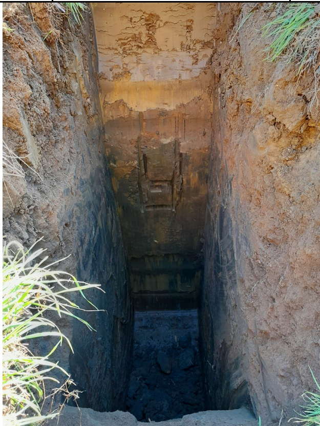
Photograph 7: TP03, dug within the embankment slope.
