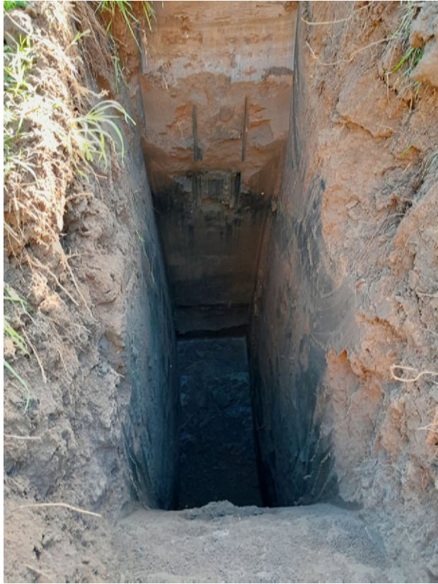
Photograph 5: TP02, dug within the embankment slope.
