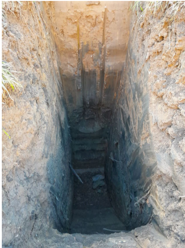
Photograph 13: TP06, dug within the embankment slope.
