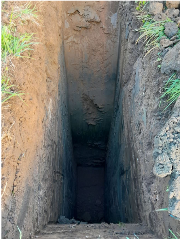
Photograph 3: TP01, dug from the top of the embankment platform.
